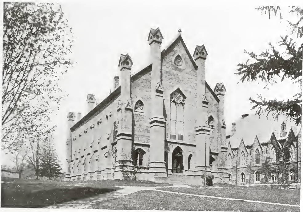
RICH HALL—LIBRARY (1866-8), WESLEYAN UNIVERSITY. Middletown, Conn. Austin & Brown, Architects.
